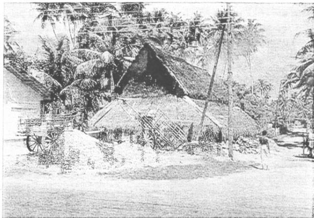
Coral mining from the sea has caused massive coastal erosion in south and southwestern Sri Lanka. Corals are burnt in kilns to produce lime. Photo: M.C. Öhman.
